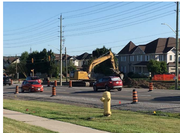
Figure 13: Brock Street widening construction, Whitby (Source: Region of Durham Planning and Economic Development Department)
